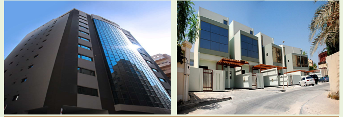
12 Storey Building in Juffair
